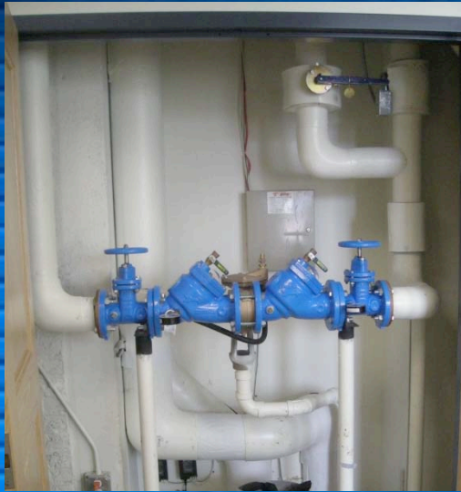
Rainwater Backflow Preventer
